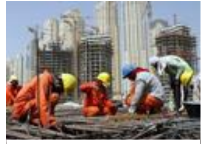
New building being built in the UAE
